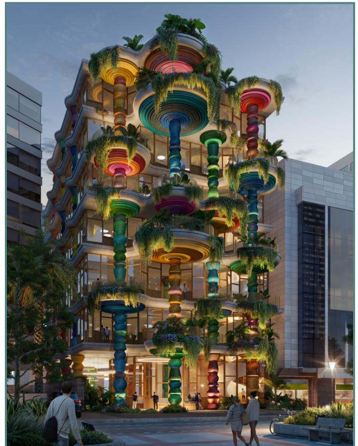
Figure 111: Public space & façade design (rendering) for Universidad EAN in Bogotá, Colombia by Heatherwick Studio; Image credit: NOD/Heatherwick Studio via ArchDaily
