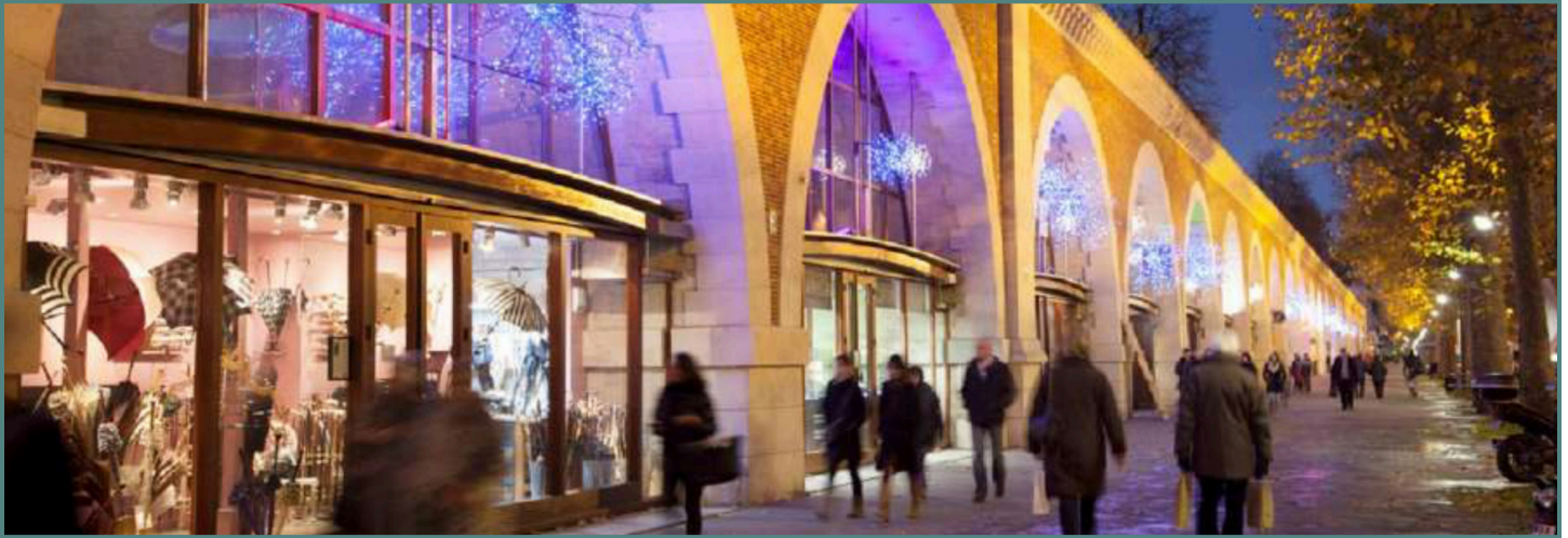
Figure 160: Viaduc des Arts, Paris; Photo credit: ©Alamy via Under the Viaduct (ARUP)
