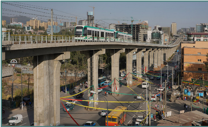
Figure 162: Addis Ababa's Light Rail, Ethiopia; Photo credit: Alexander Savin, WikiCommons
